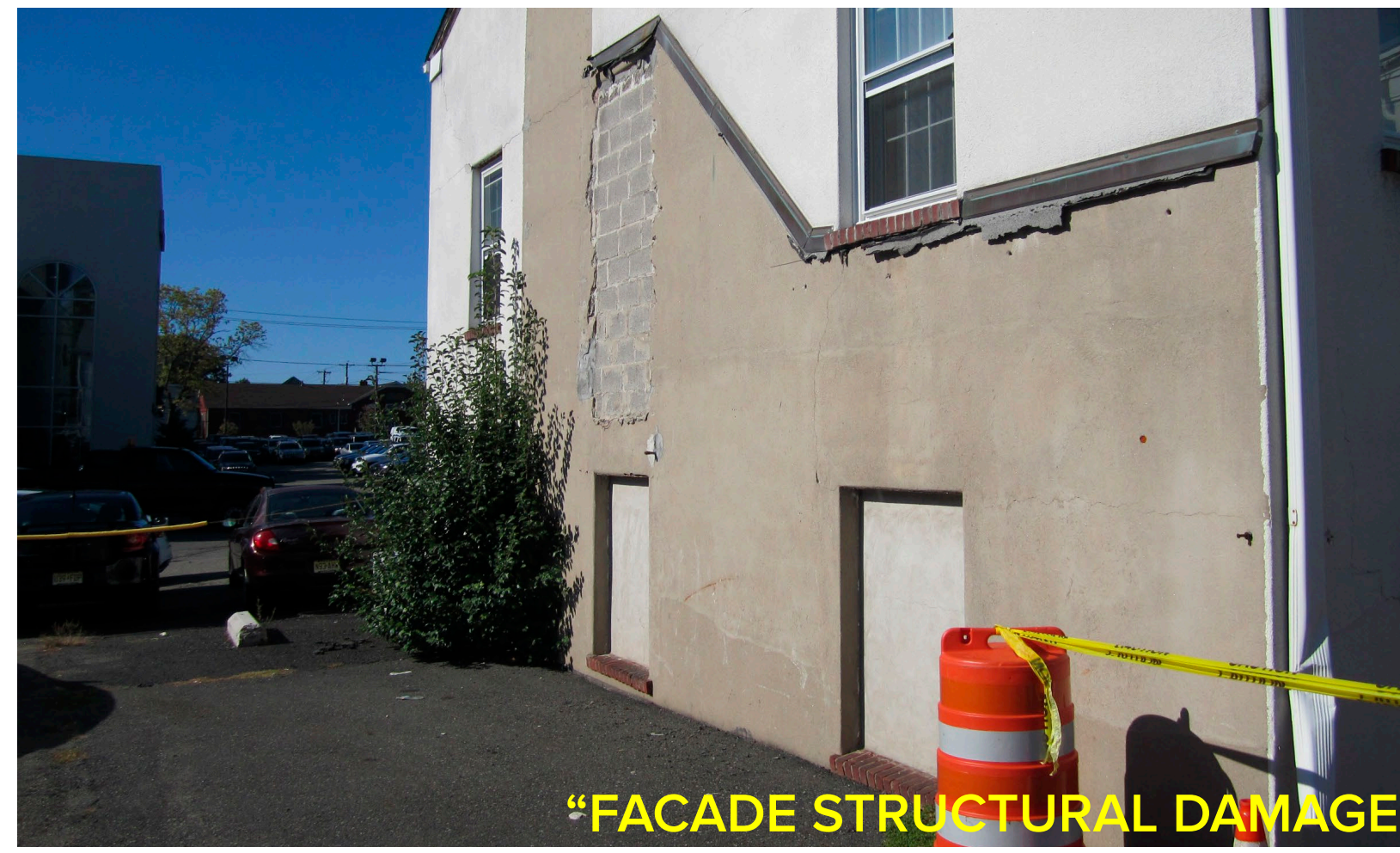
"WATER DAMAGE - STUCCO - CAN SEE DAYLIGHT"
