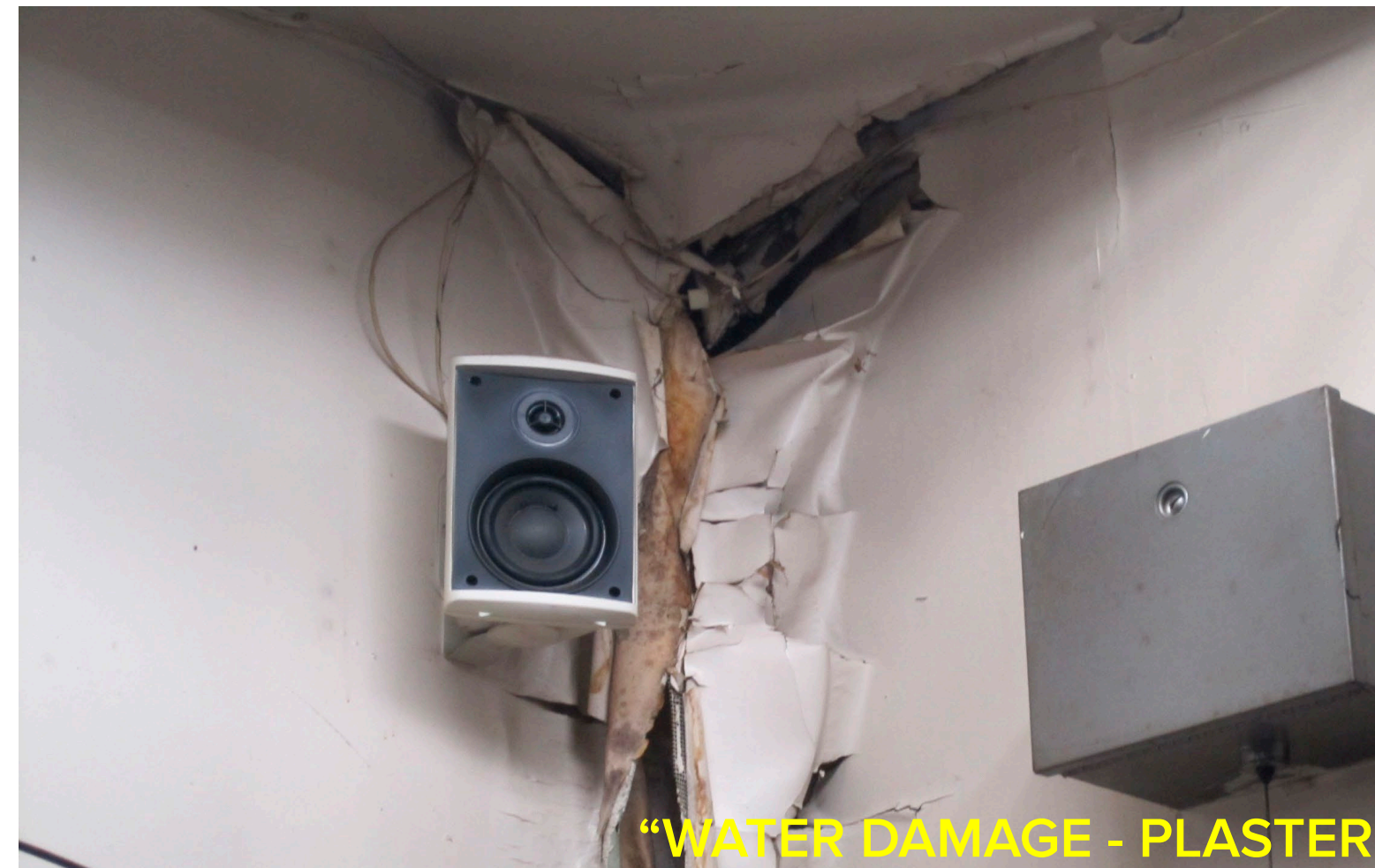
“WATER DAMAGE - PLASTER”
